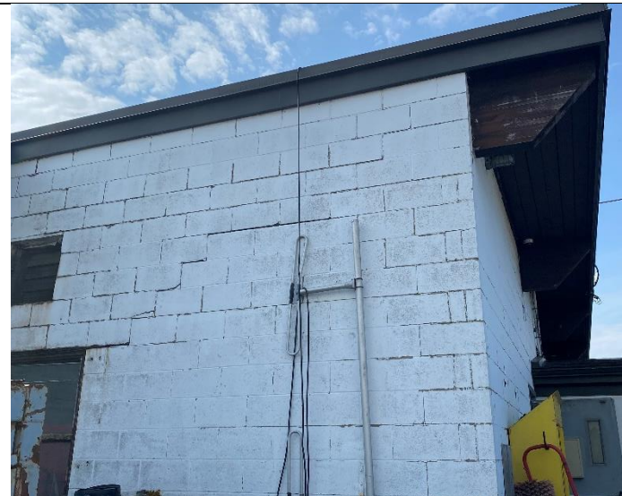
Photograph No. 51) Step cracking in CMU wall at North-West corner.
