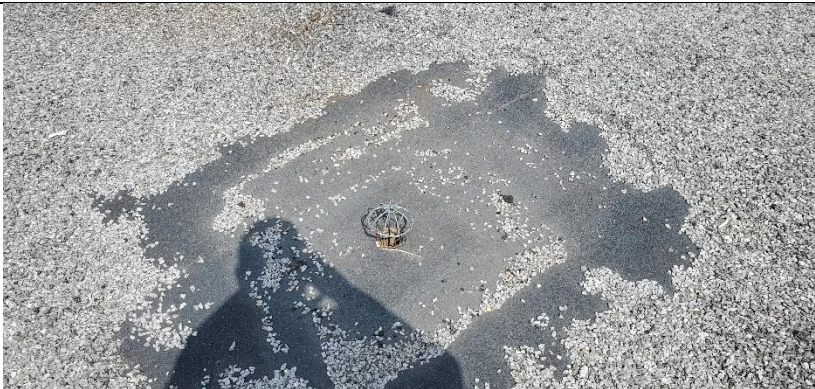
Photograph No. 3) Three of four roof drains need a proper cover.
