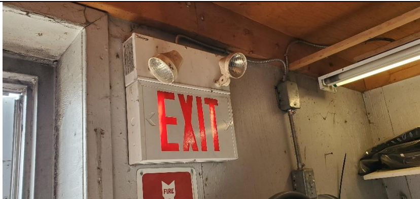
Photograph No. 35) Illuminated exit sign with emergency dual remote head with battery pack provided in the back shop area.
