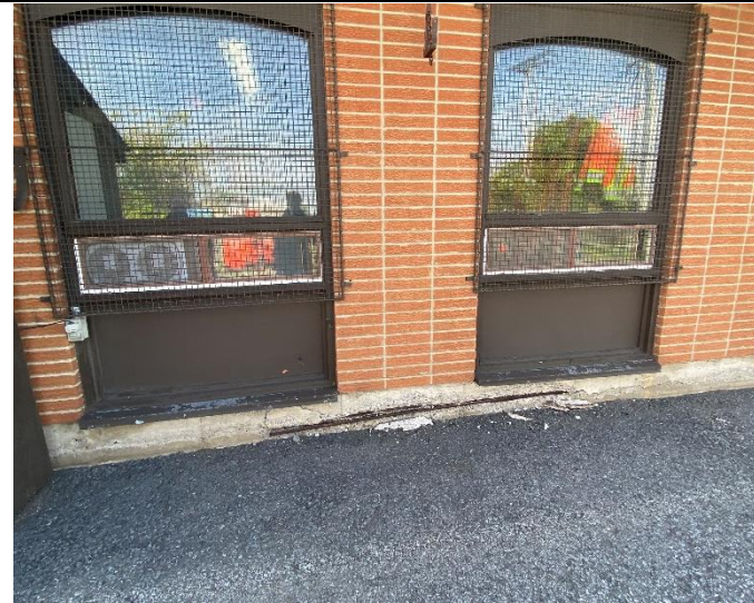
Photograph No. 53) Location of exposed rebar in top of foundation wall of the office addition.
