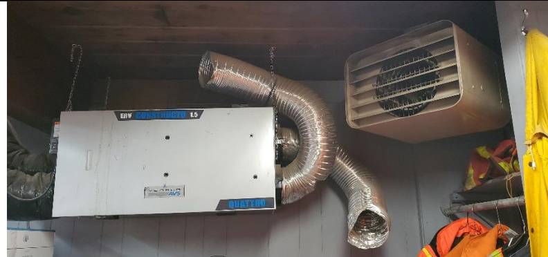
Photograph No. 18) ERV and electric unit heater provided in the change room.
