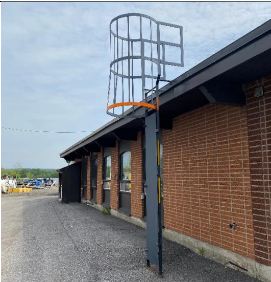
Photograph No. 58) Roof access ladder on the office addition, the condition of the pavement can be seen beyond.
