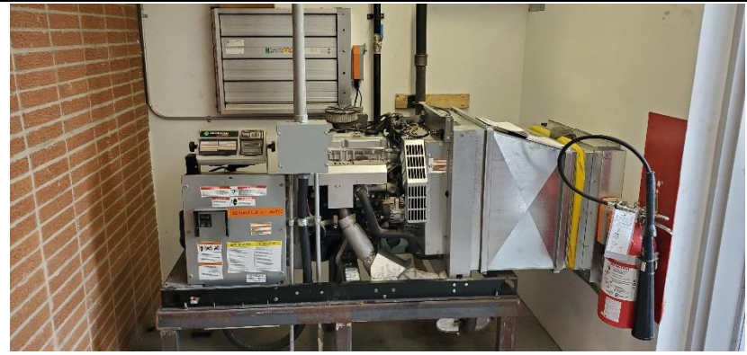
Photograph No. 38) "Generac" emergency generator provided in the generator room.
