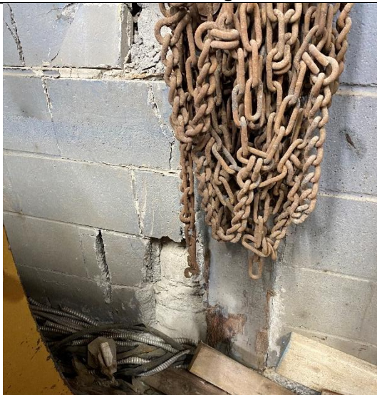
Photograph No. 50) Damage to CMU wall at back of garage.
