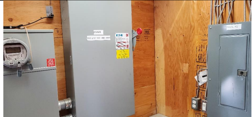
Photograph No. 26) Main transfer switch provided in the generator room.
