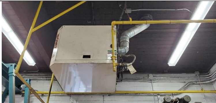
Photograph No. 19) Typical “Reznor” gas-fired unit heater provided in the garage.
