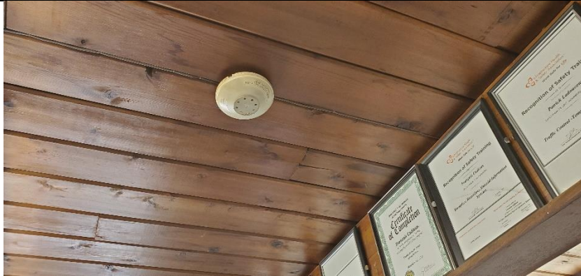
Photograph No. 37) Typical smoke alarms provided throughout the office and garage building.
