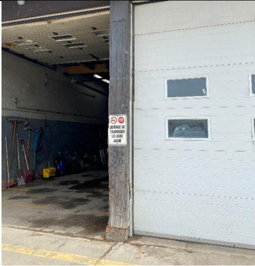
Photograph No. 48) Typical wood column supporting deep roof beam with damage.
