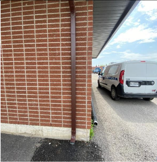
Photograph No. 60) Typical condition of the brick veneer on the office addition, and a roof gutter downspout.
