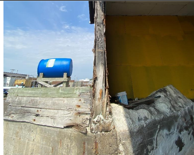
Photograph No. 57) Typical condition of the framing of the salt shed.
