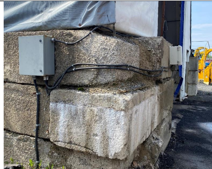
Photograph No. 55) Typical deterioration of the salt dome concrete blocks.
