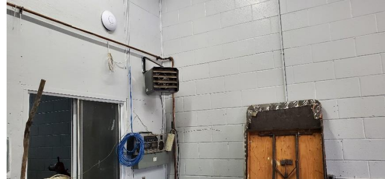
Photograph No. 42) Electric unit heater provided in the east garage area. Unit to be replaced due to low heating capacity.
