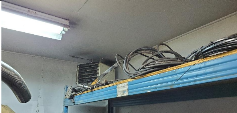
Photograph No. 41) Electric unit heater provided in the back storage area.
