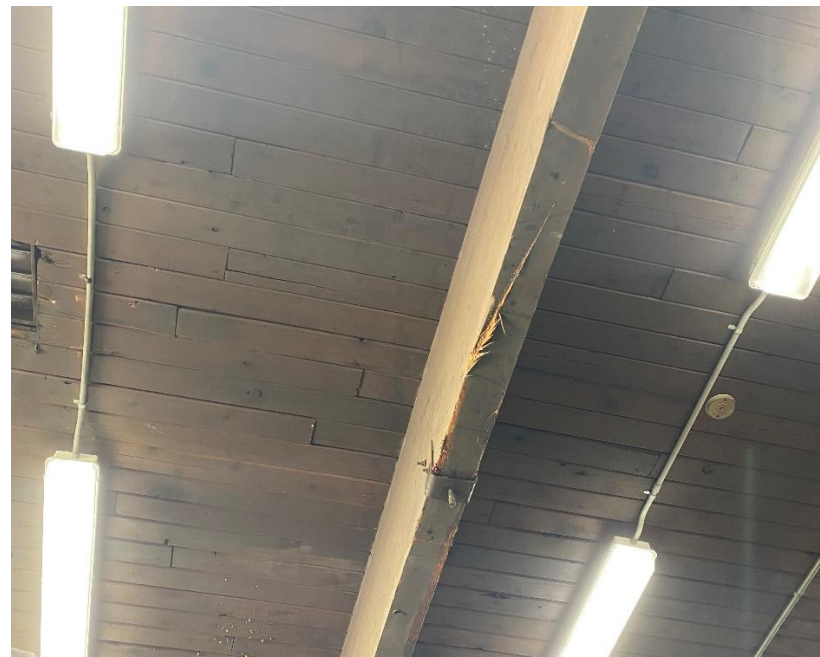
Photograph No. 47) Typical damage to the deep glulam beams from equipment strikes.
