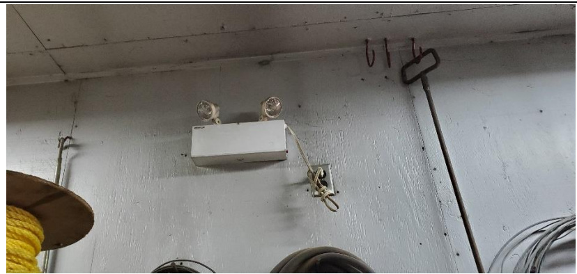
Photograph No. 36) Emergency dual remote head with battery pack provided in the back shop area
