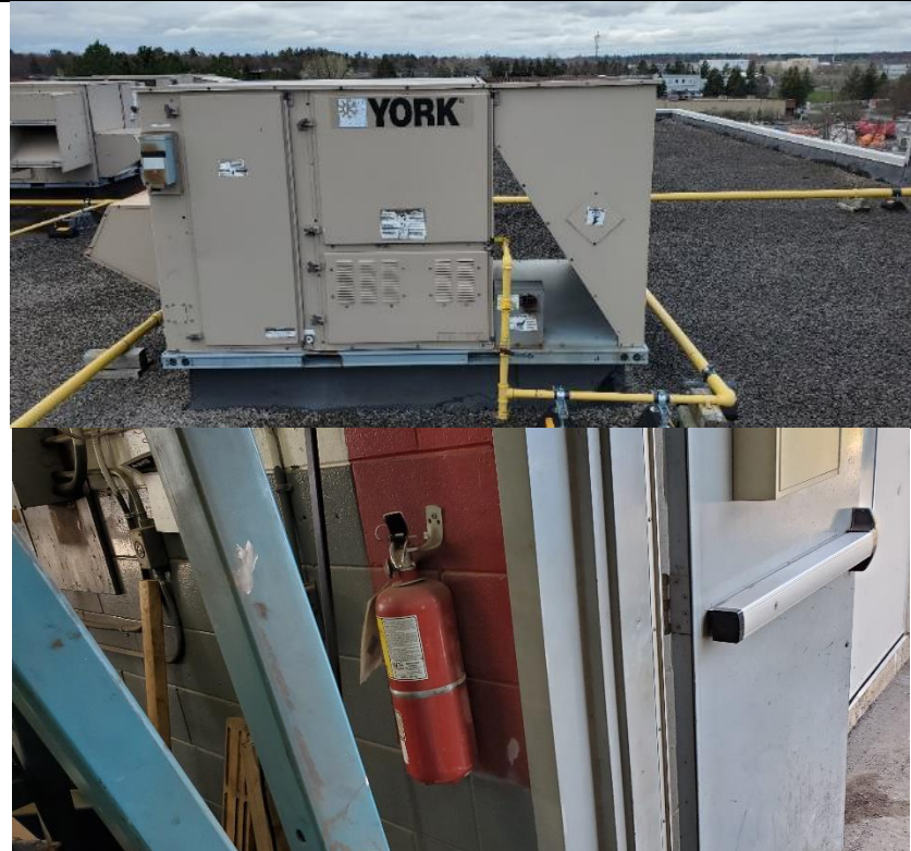
Photograph No. 24) Typical ABC type portable fire extinguisher provided throughout the office and garage.
