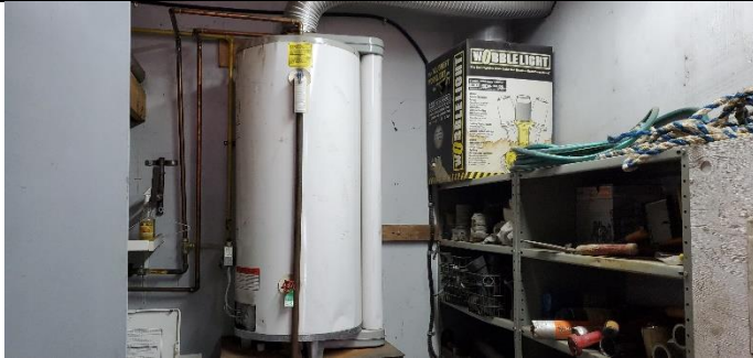
Photograph No. 5) "GSW" gas-fired hot water heater provided in the back shop area.
