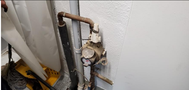
Photograph No. 1) Domestic water entrance provided in the office washroom.
