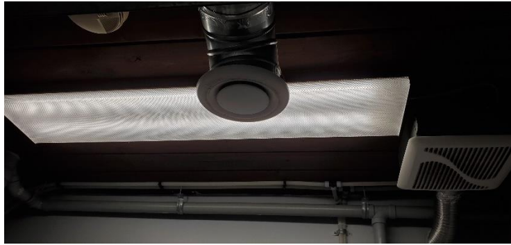
Photograph No. 17) Exhaust fan provided in the office small washroom.
