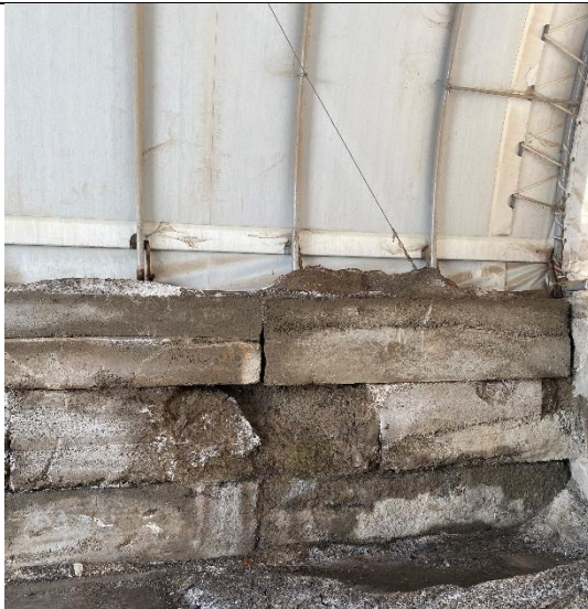
Photograph No. 54) Typical deterioration of the salt dome frames and foundation.
