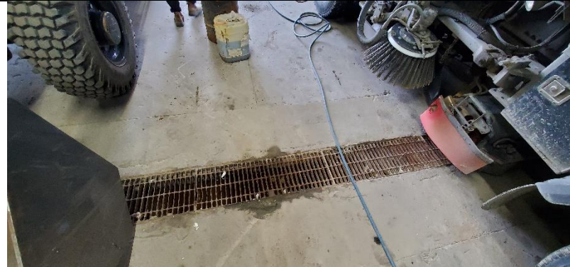
Photograph No. 14) Typical trench drain provided in the garage.
