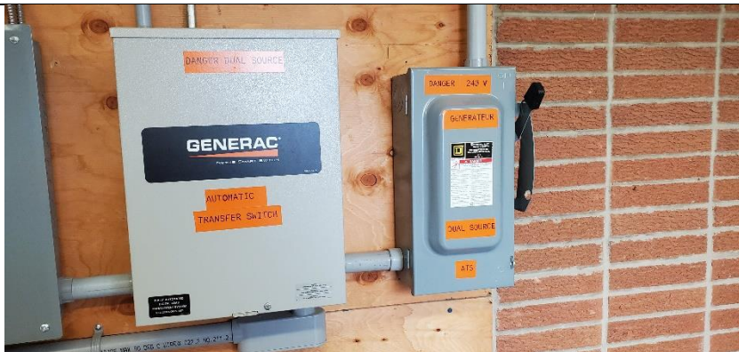
Photograph No. 39) Automatic transfer switch for generator provided in the generator room.
