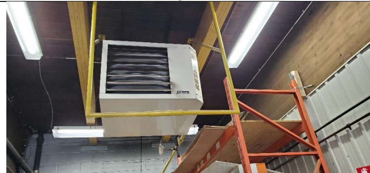
Photograph No. 20) Typical “Reznor” gas-fired unit heater provided in the garage.
