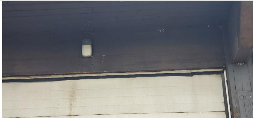
Photograph No. 32) Typical fluorescent wall mounted exterior light fixture provided on the perimeter of the office and garage building.
