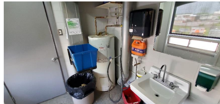
Photograph No. 4) "Giant" electric hot water heaters in the office washroom.
