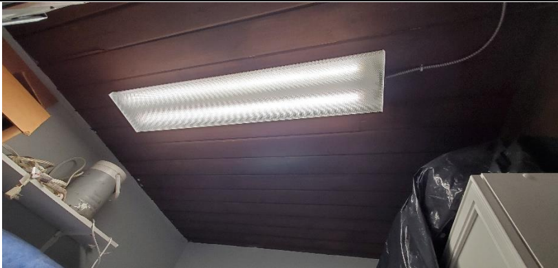
Photograph No. 29) Typical fluorescent 1'x4' ceiling light fixture provided throughout the office.
