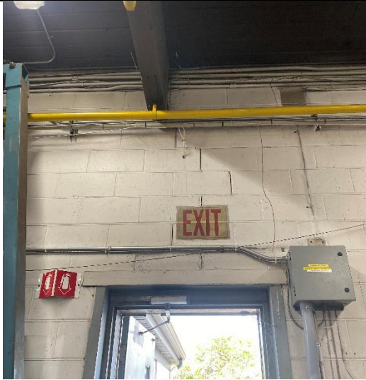
Photograph No. 52) Step cracking in CMU wall below beam support.
