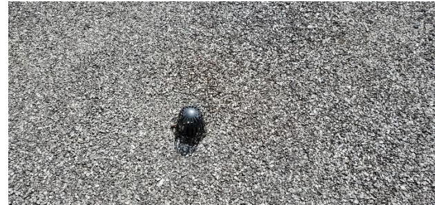
Photograph No. 2) Cast iron roof drain provided on the garage roof.
