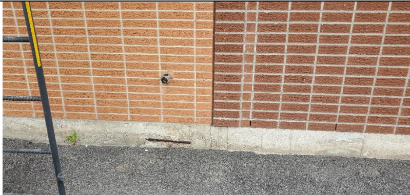
Photograph No. 15) Hose bib provided on the exterior of the office building.
