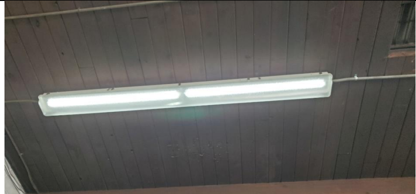
Photograph No. 30) Typical fluorescent strip light fixture provided throughout the office, generator room and back storage area.
