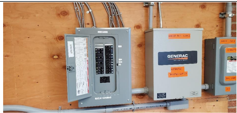
Photograph No. 28) Emergency electrical panel provided in the generator room.
