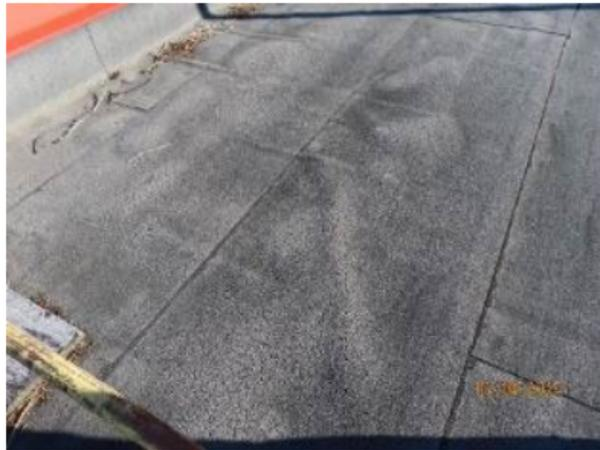
B3010-2 - View of modified bitumen roof with noted wrinkles.
