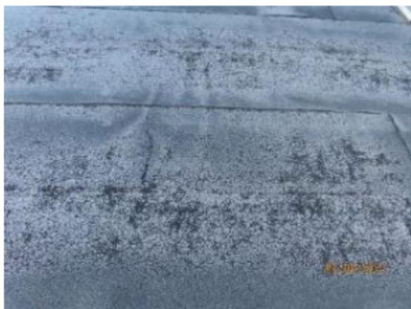
B3010-5 - View of deteriorated bitumen modified roof.
