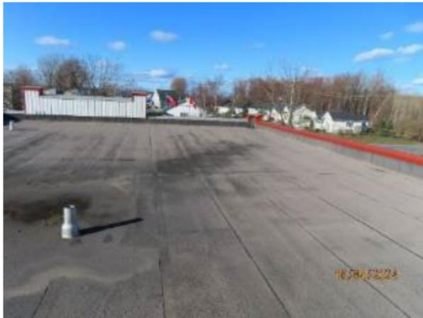
B3010-1 - General view of 2-ply modified bitumen roofing system.
