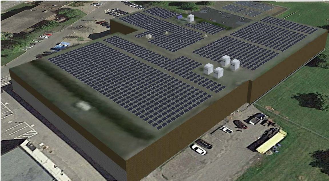
Figure 9: Rendering of a 380 kW roof top solar array on the Robert Hartley Sports Complex.
